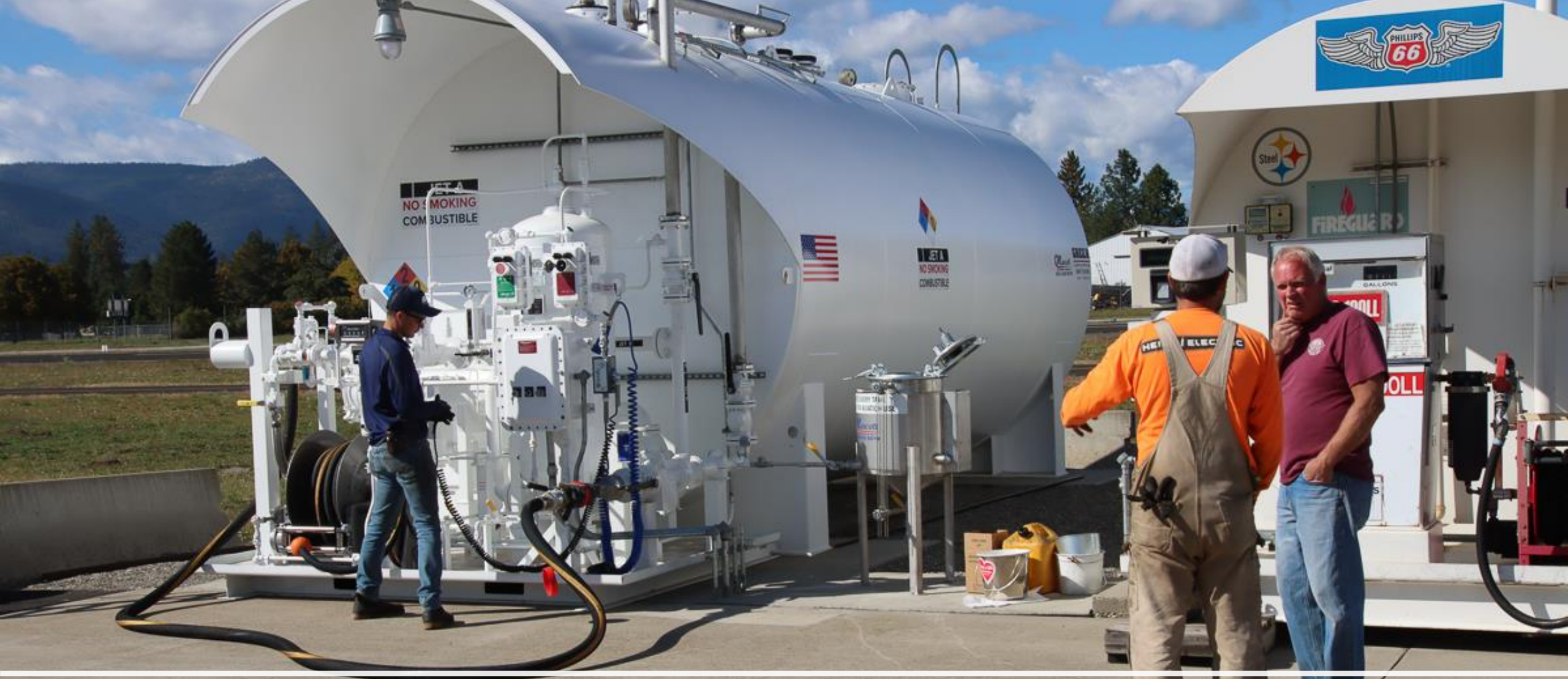
The Fuel Tank's Final Installation
